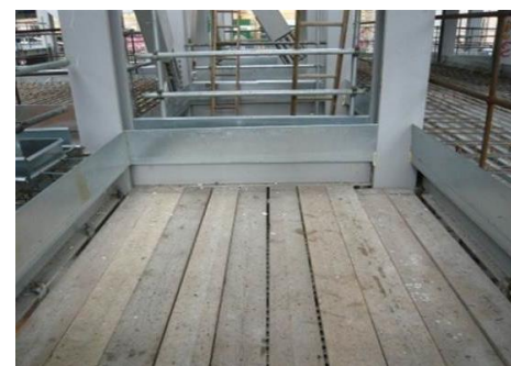
Figure 2. Scaffolding used as a working area for metal decking
